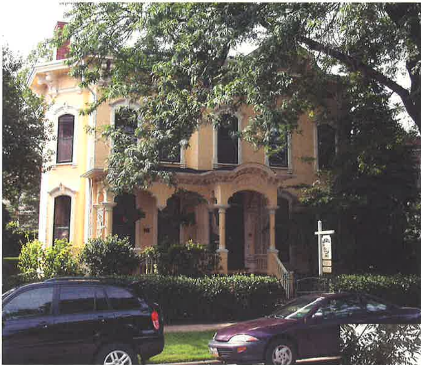
Bevelin House at 2913 Clinton Avenue dates from the 1850s.
